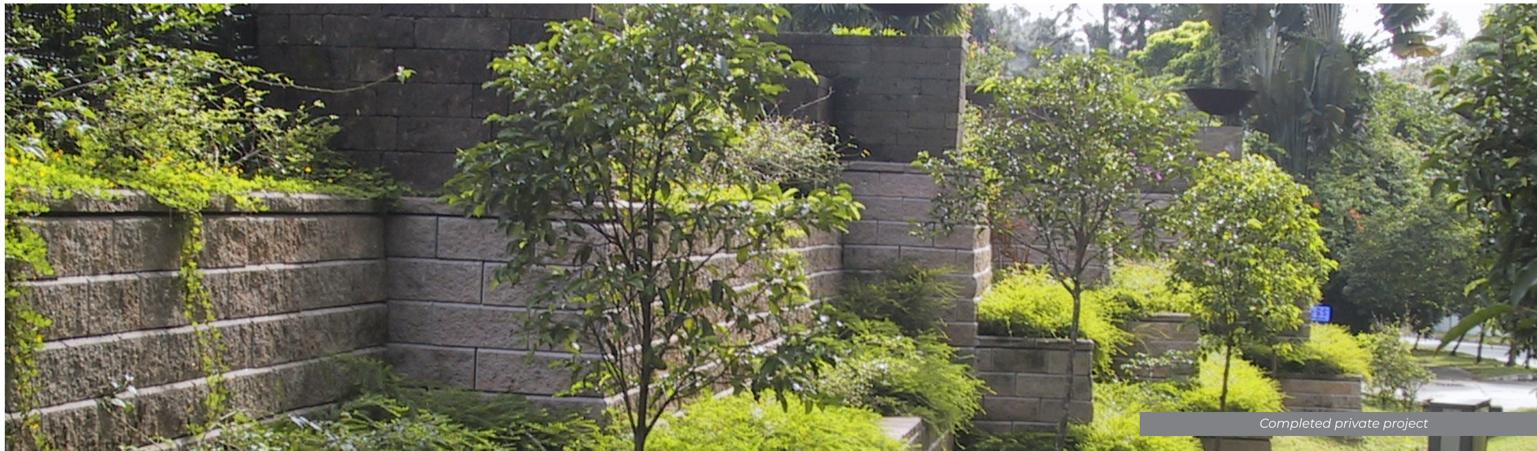
Completed private project
