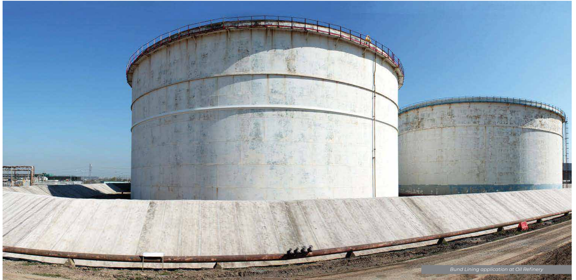
Concrete Canvas used for drainage
